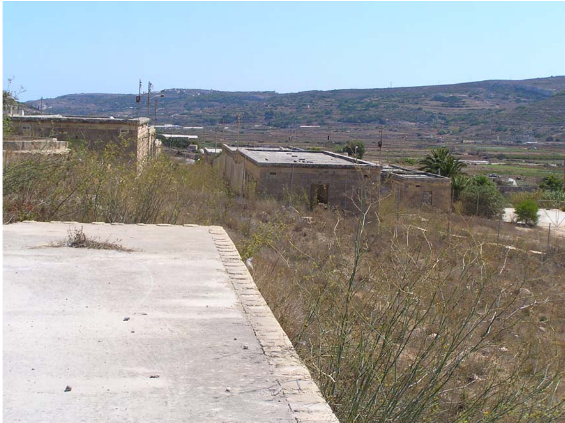
Image 3: Barracks built at different levels along slope
