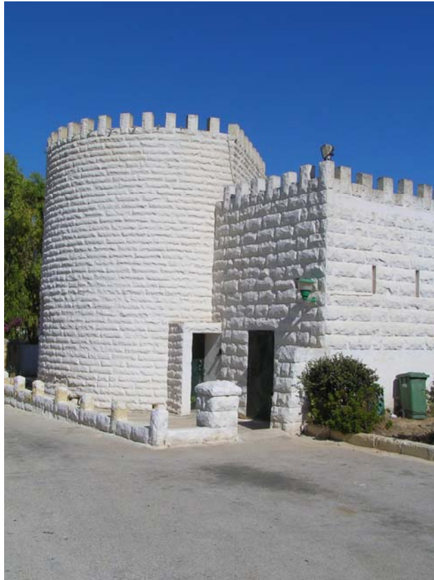
Image 13: Building from 1970s near Entrance (C18)
