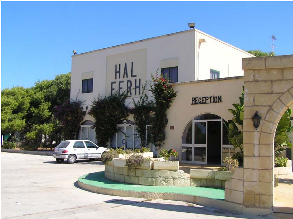
Image 11: Reception Building of Holiday Complex (C15)
