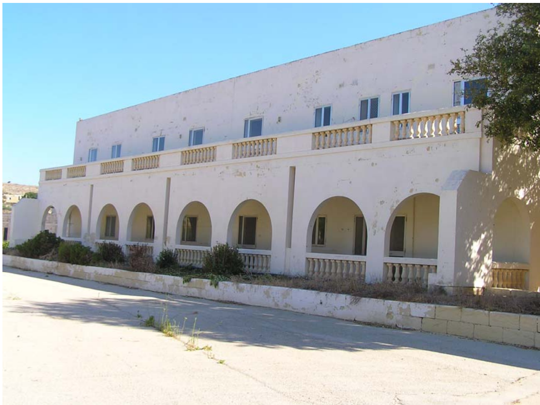
Image 12: Large Building built in 1980s (C11)
