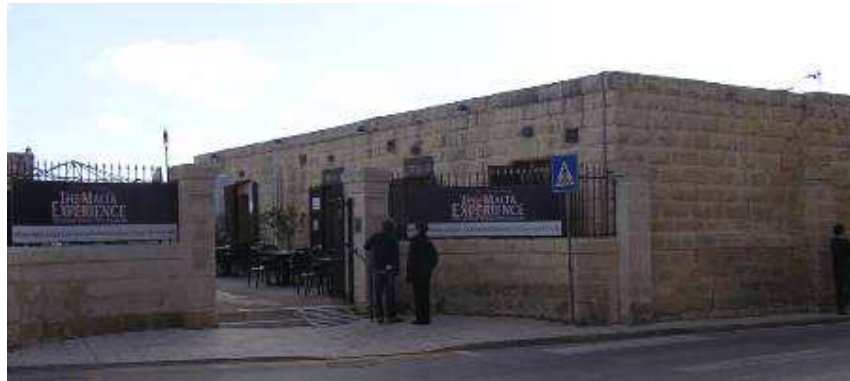
Image 9: The Malta Experience building
