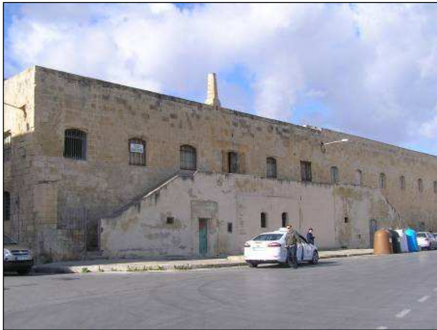
Image 14: Examination Centre front elevation
