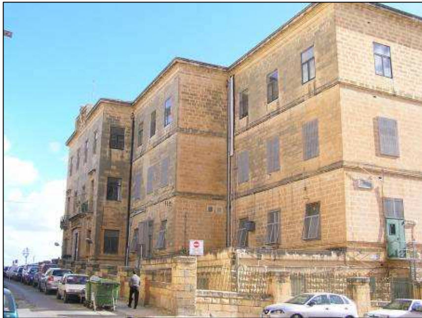
Image 12: Evans Building elevation from Triq il-Merkanti
