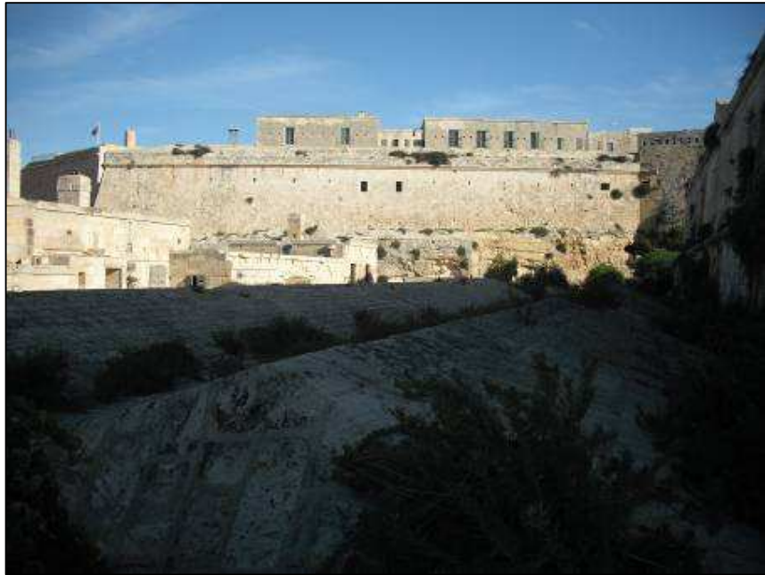
Image 6: Roof of bomb-proof Vendome water tank structures
