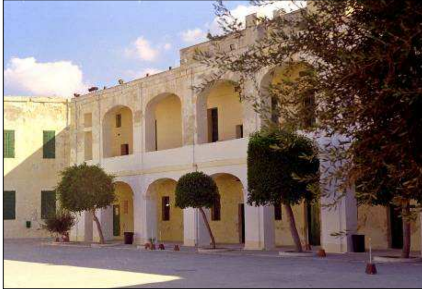
Image 3: Barrack building within Fort St. Elmo
