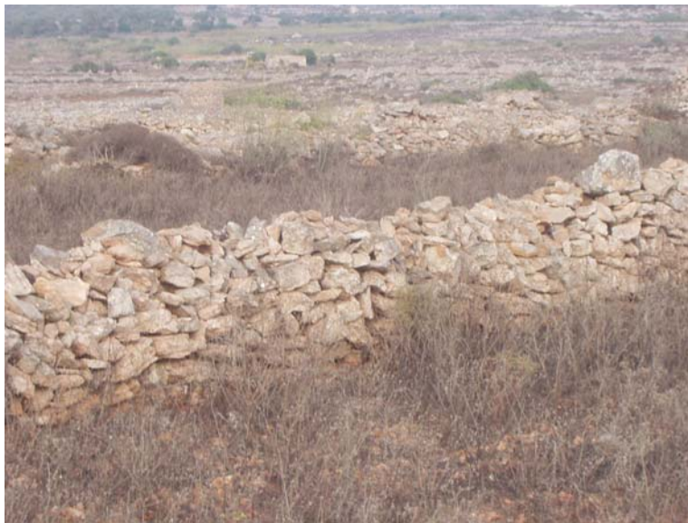
Figure 6: Grade A rubble wall
