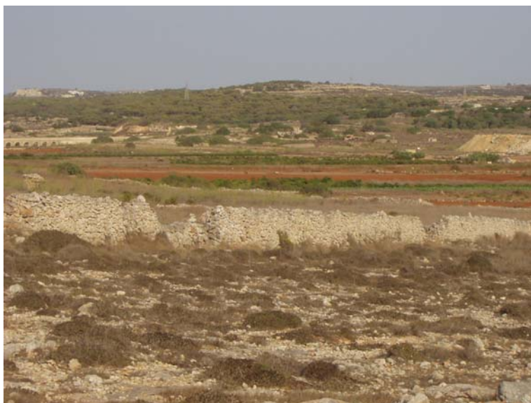
Figure 7: Grade B rubble wall
