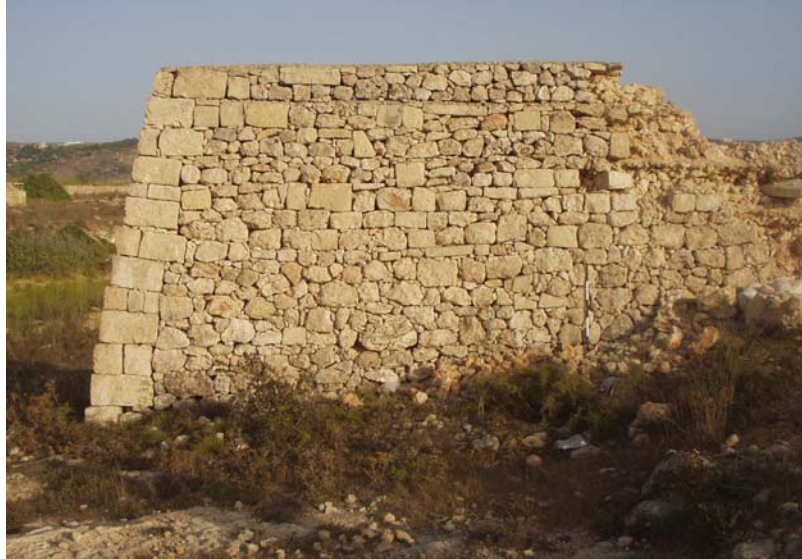
Figure 21: Entrenchment MNK05_094 similar in construction to the technique shown in Figure 12
