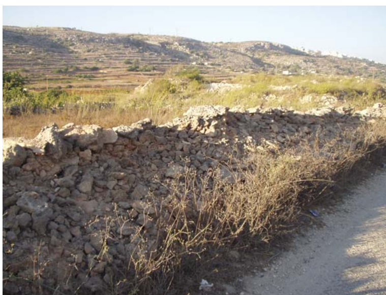
Figure 8: Grade C rubble wall
