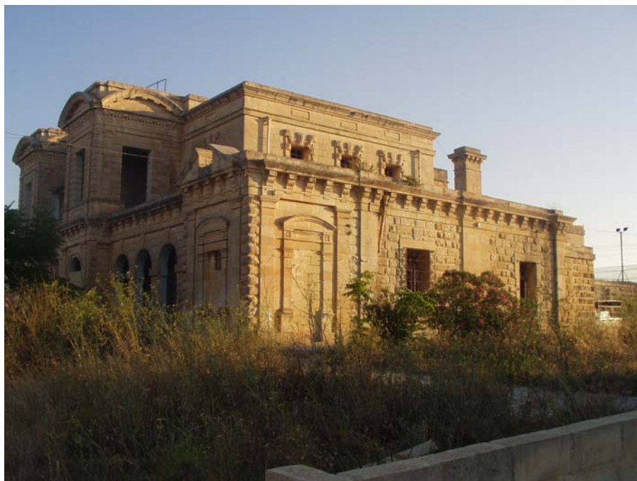
Figure 12: 82/583/96, Derelict Ex-Raffles Discotheque at Triq Arnhem, Pembroke
