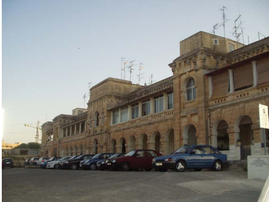
Figure 9: 93/583/96, Ex-Barracks Block No.3 Flats 1-10 at Triq Falaise , Pembroke
