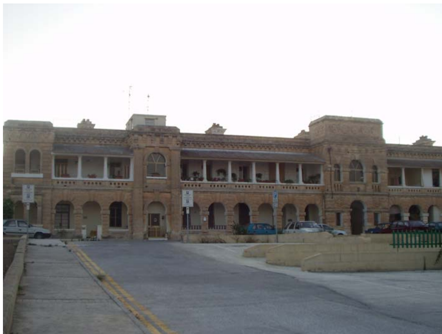
Figure 6: 92/583/96, Ex-Barracks Block No 2 Flats 1-10 at Triq Suffolk, Pembroke
