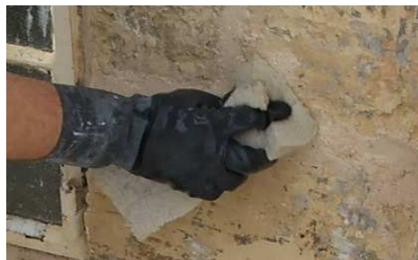
Pointing using a mortar piping bag
